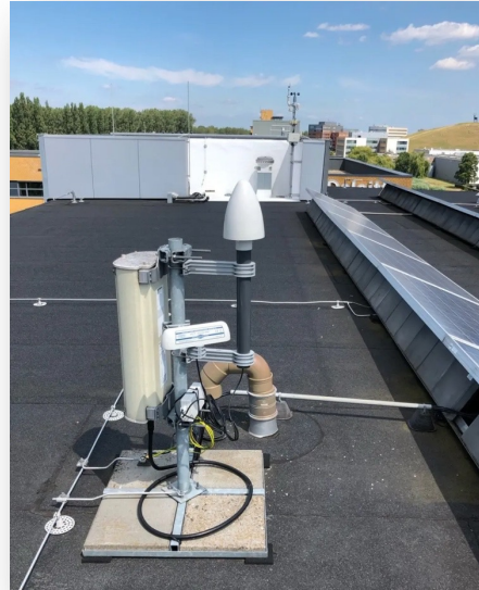
Provide well-managed and secure time services
